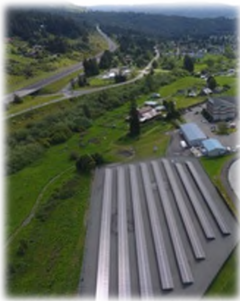
Microgrid solar array at Blue Lake Rancheria. Credit: BLR
