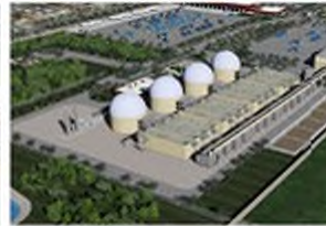
Anaerobic Digestion Facility - ADF
