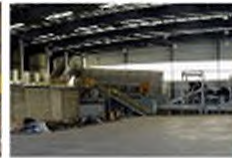
Organics Receiving Facility - ORF
