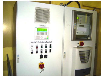
Figure 2-3: SCR Control System
