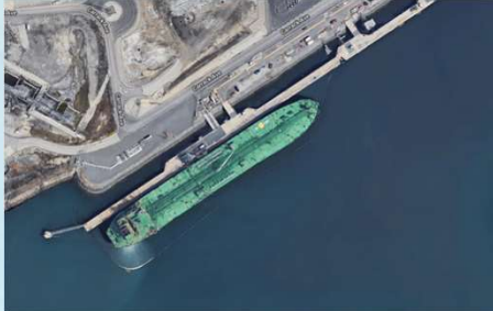
Tanker terminal at Port of Long Beach
