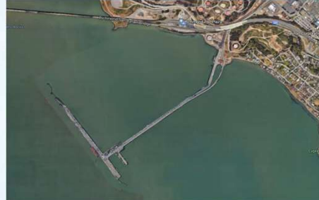
"T"-shaped marine oil terminal in Northern California
