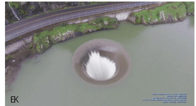
Monticello dam spillway
