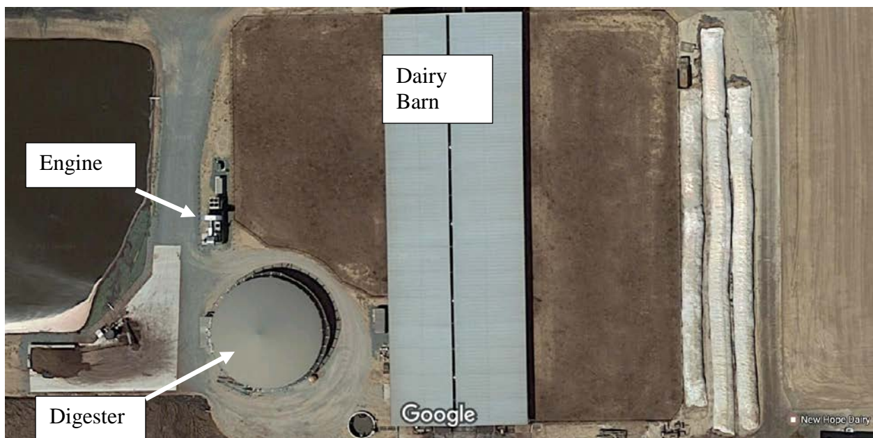
Figure 2-4: Over-view of New Hope dairy biogas production facility.
