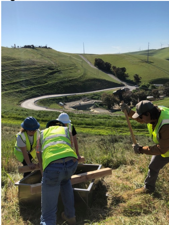
Figure 3.7 Installation of Chamber Collar
