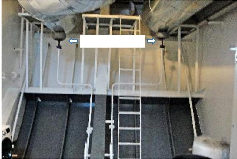
Team members from the University of British Columbia worked with the vessel operator to remove the valve from the KO system and added a blank flange with four connections to the sampling lines, as shown in Figure 2. A transfer line was built from the exhaust to the dilution tunnel. The same dilution tunnel was used throughout the project to ensure a consistent dilution ratio for all test results.
