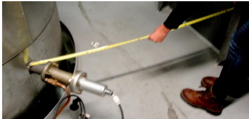
Figure 2-4 Platform space available for equipment (smoke meter shown)
