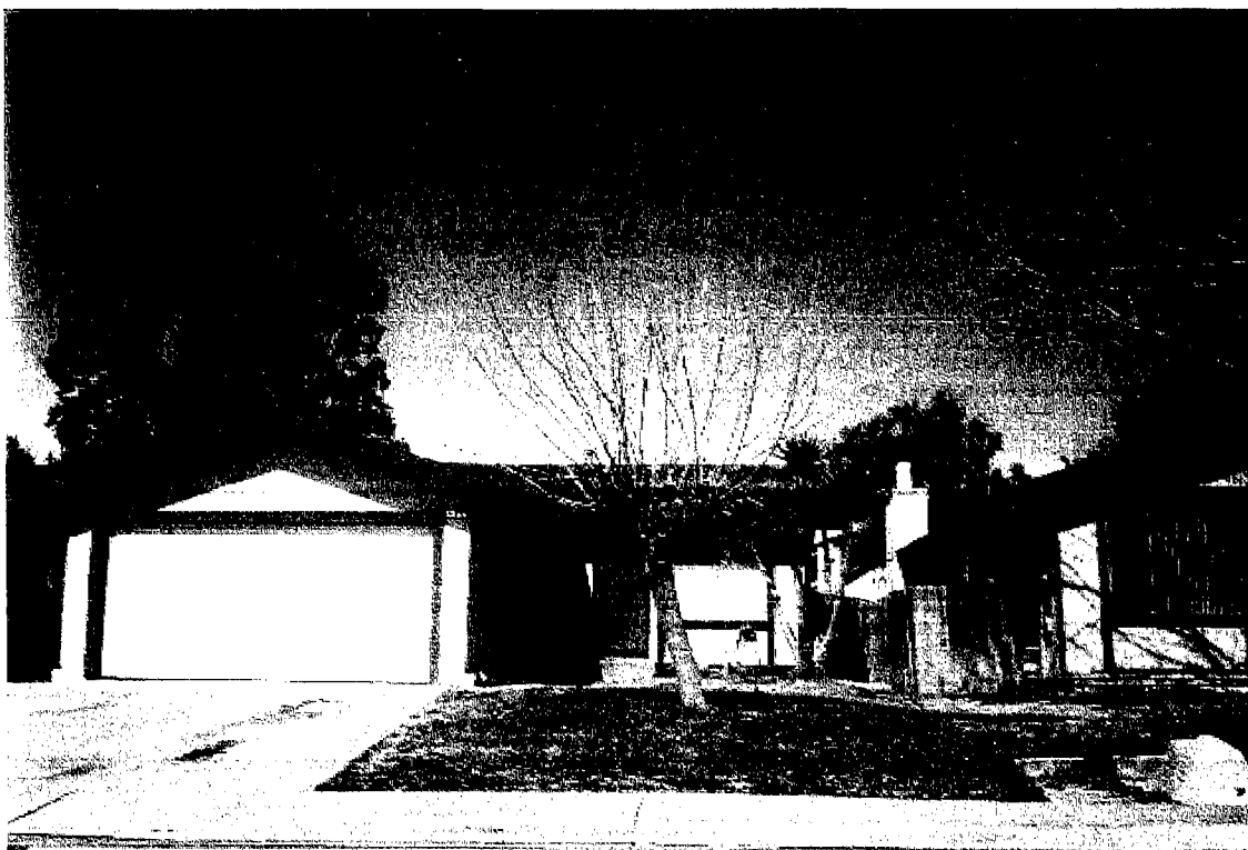
Figure 2-2. Front Elevation of the Test House
