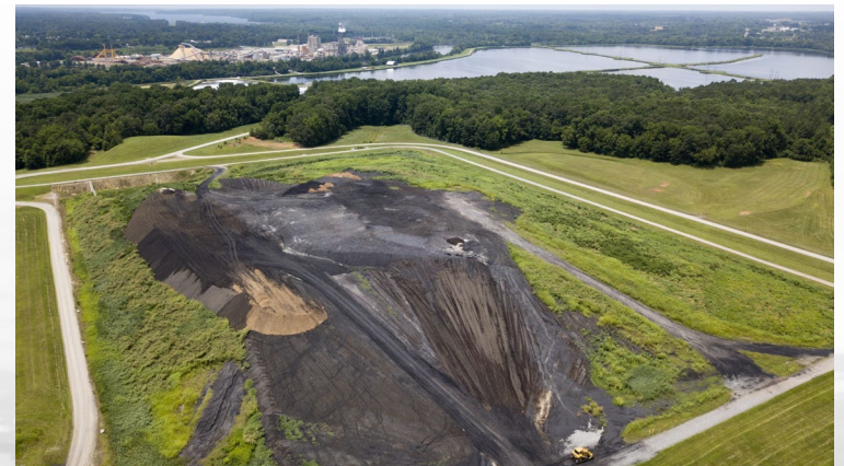
Reclaimed Fly Ash
